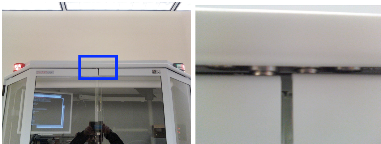
Figure 1: Bolts and washers that hold X-Ray door on rail. Picture on Right is enlarged view of the part in the blue box.
